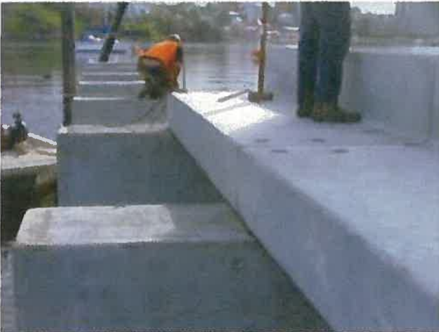
Photo C: View along pile caps showing fixed panels in place.
