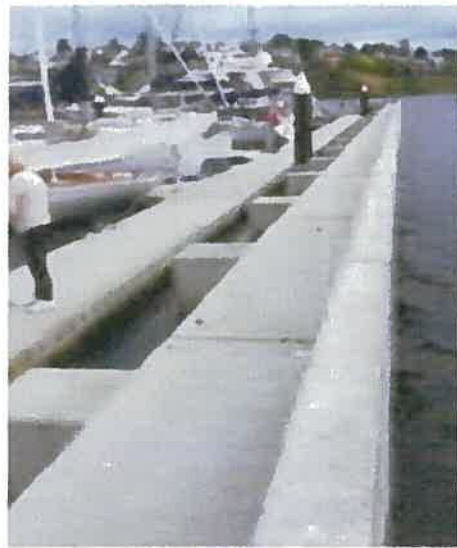
Photo D: View of completed wave attenuator and floating marina.
